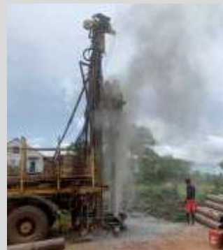
Sierra Leone: Water borehole for school complex
