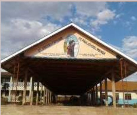
Tanzania: Construction of an Open-Air Pavilion at De Paul School
