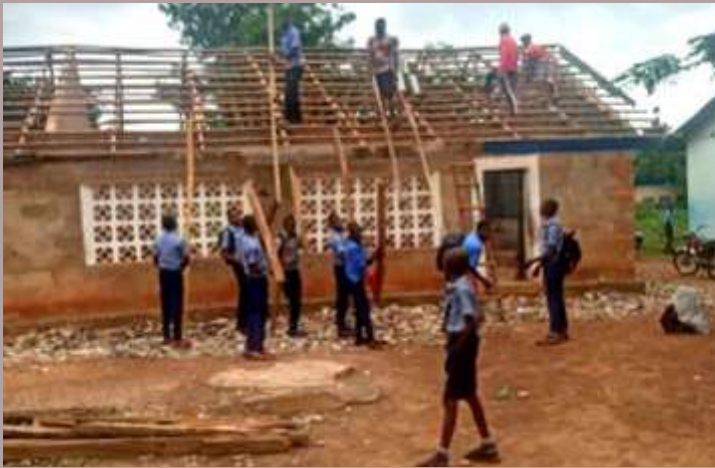
Nigeria: Roofing Of St. Mary's College Multi-Purpose Auditorium
