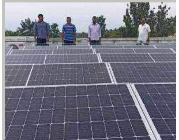
Fr. Anil Thomas CM, Fr. Jijo Joseph CM, Fr. Tibin Mathew CM, and Fr. Stephen Antony, CM of the South India Province on the roof of the provincial house with new solar panel bank installed.
